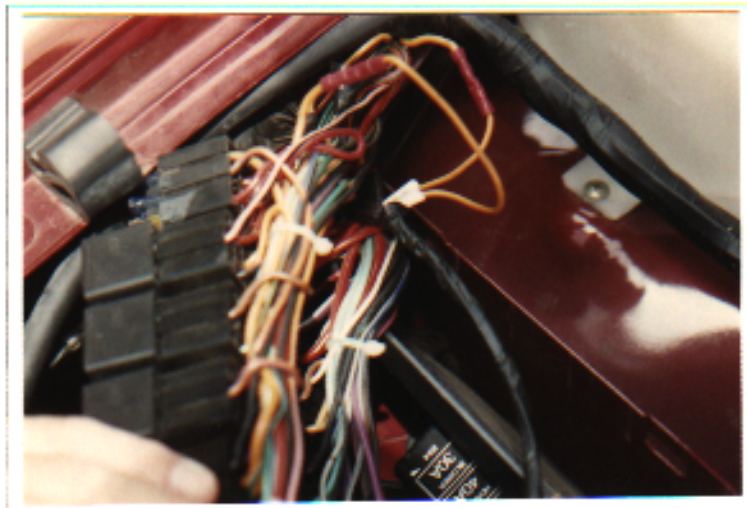
Fig. 11 Relay Bar Removed From Mount Showing Isolation splice
